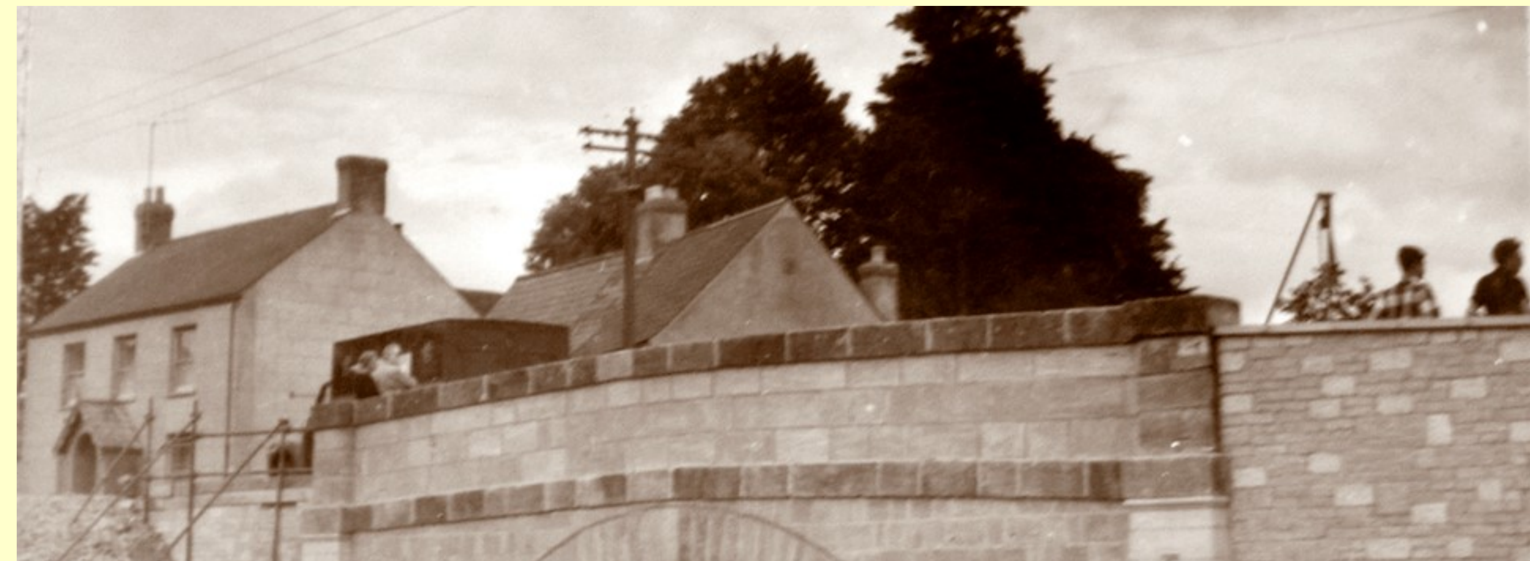
In 1957 a new bridge was built, the Charmouth men assisting in the building were :- E. Harry Grinter, Fred Grinter, Alfred T. Bradford, Brian Bowditch and Charlie Stirk . The crown was lowered by 2 feet 9 inches which gives a clear sight line and a smooth gradient.
