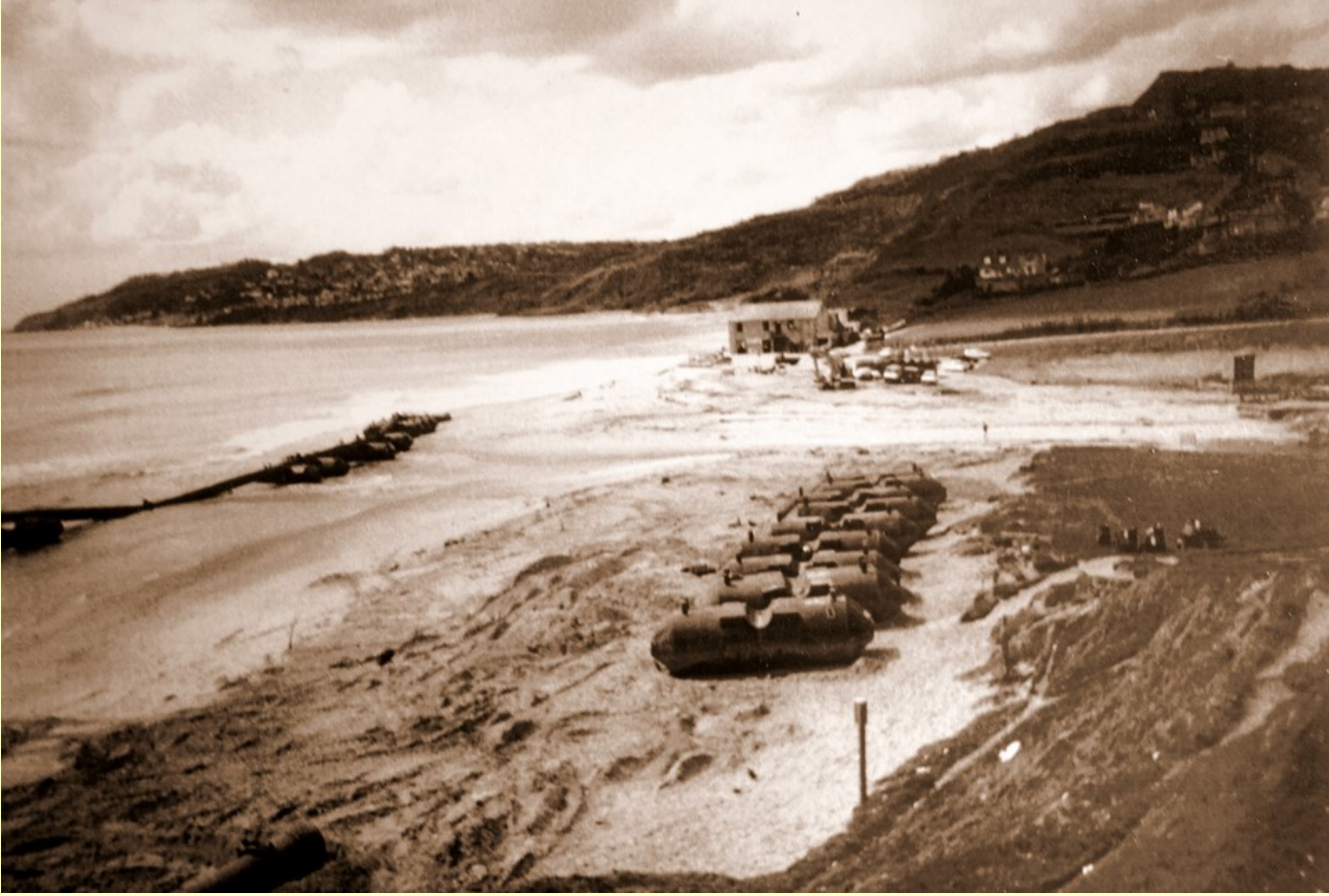
The Sewage pipes are seen here in the process of being laid out to sea.
